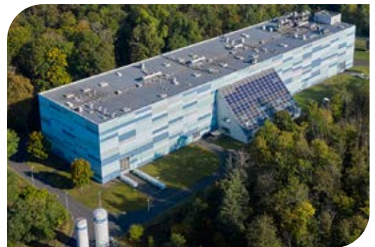
Fig. 1: The Aschaffenburg water treatment plant
