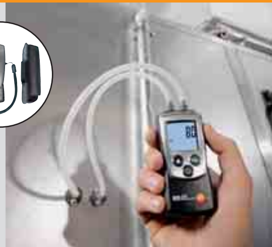
Differential pressure measurement on filters
